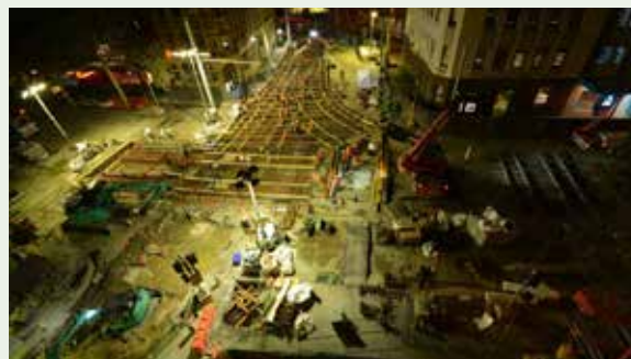
Figure 37: The use of temporary lighting systems must avoid loss of amenity within the local neighbourhood. This can be achieved through selecting and positioning lighting systems that minimise or prevent light-spill and glare.
