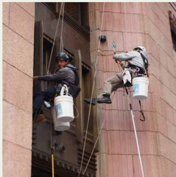
Figure 26: Rope access ( hoisting activity) to undertake minor maintenance activity e.g.: window cleaning, is permitted subject to approval being given to establish exclusion zones (see Figure 25 ). The PCBU must risk assess this activity and implement any necessary control measures . All ropes are to be contained within the pedestrian exclusion zone (barricaded space).
