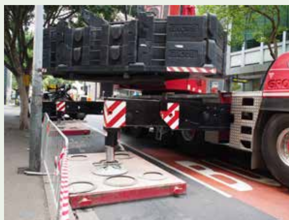
Figure 2: Bearing pressures transferred through outriggers must be evenly distributed to prevent damage to roadways . Outriggers and crane bodies must not encroach on through-traffic lanes that are required to be kept open.
