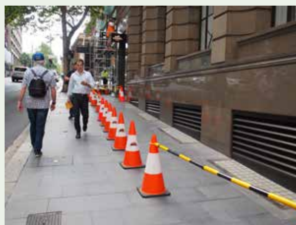
Figure 16(a): Temporary barricading must minimise impacts and maintain safe and convenient pedestrian passage. In some cases barricading will not be permitted during the peak pedestrian periods. In very busy areas such as shopping districts, works and barricading may need to be undertaken at night or on weekends.
