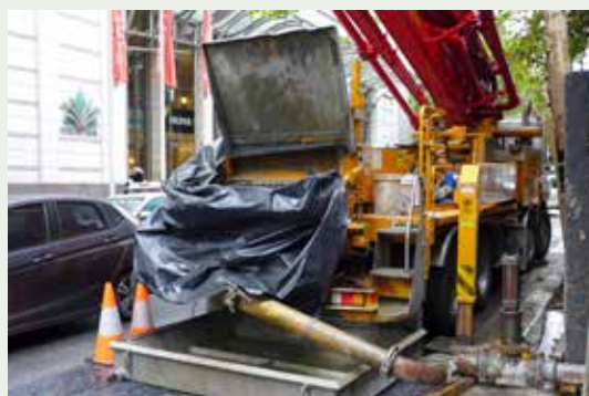
Figure 18: Pollution prevention measures must be in place during concrete pumping operations to prevent spillage onto roadway surfaces and pollution offences (stormwater pollution).
