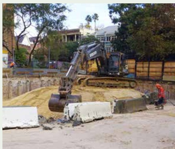
Figure 47: The short-term stockpiling of excavated material that is awaiting removal from a site is permissible subject to specific approval being given. Effective environmental and amenity controls must be implemented including measures to prevent the movement of material in water run-off and through wind actions.
