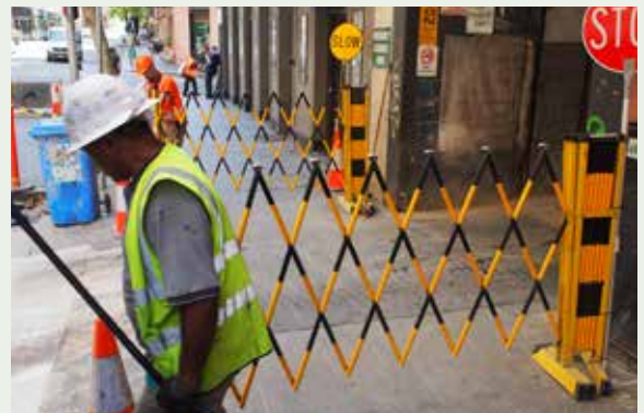
Figure 43: The effective control and safety of pedestrians and cyclists at truck access points is essential. This is particularly important in high volume pedestrian areas. The City will allow, and require, the use of manned concertina gates as a control measure .
