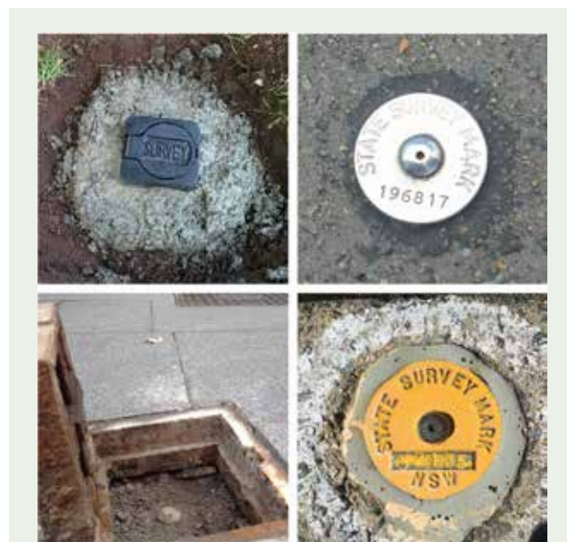
Figure 48: Examples of survey marks located in the City of Sydney LGA. Survey marks are important survey assets and are protected under legislation.
