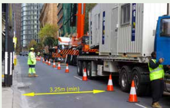
Figure 6: Where required by the City a clear 3.25 metre traffic lane must be provided and maintained during a partial road closure.
