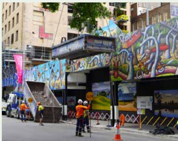
Figure 34: Through-traffic must not be stopped during hoisting operations from a road . For wide loads (greater than 2.4 metres) traffic can be temporarily stopped for a short duration until the load has reached a height of 4.5 metres above the roadway (subject to meeting prescribed requirements of this Code and approval ).
