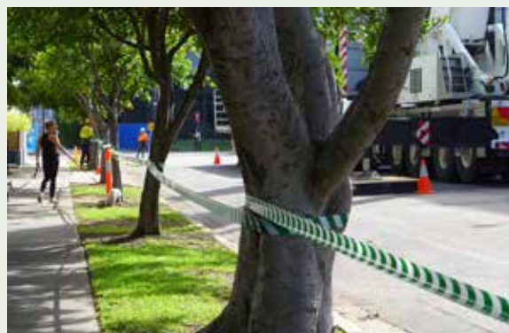
Figure 7: Appropriate barriers must be installed to isolate an approved work/crane operation area. In busy pedestrian areas such as the city-centre, metal barriers must be used.
