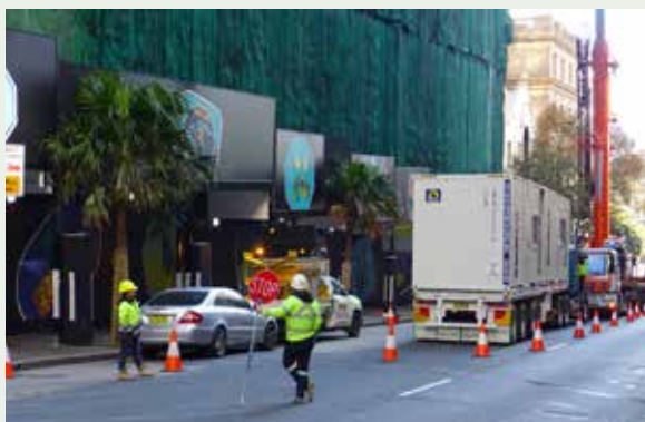
Figure 8: Through-traffic lane/s adjoining a work place must be supervised by authorised traffic controllers.
