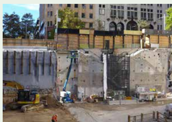
Figure 45: Shoring and ground-anchoring placed within the road reservation to support roads adjoining excavations require the approval of the City . Excavations must also be protected using appropriate pedestrian and traffic barriers (see 4.5.3 )
