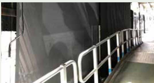
Figure 19: The use of screens to protect pedestrians and cyclists from concrete over-splash at pumping locations is generally not supported by the City . Where approval is given temporary screens must be of a durable quality, satisfactory design and fixed securely in place. Screens must be removed from the public space immediately following completion of daily pumping operations. The City may allow screens such as roller blinds to be fixed to a hoarding (with blinds rolled up when not in use to allow unimpeded pedestrian access at the kerb).
