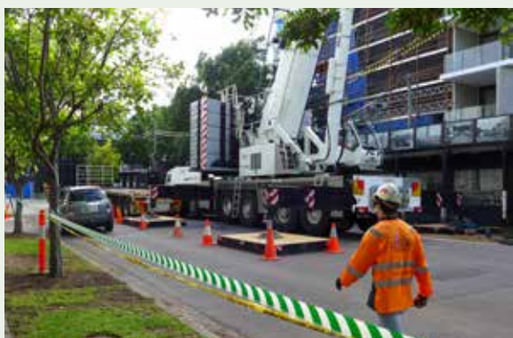
Figure 9: Where approval is given to establish and operate hoisting devices on roadways , special controls will need to be implemented including traffic/pedestrian control measures .
