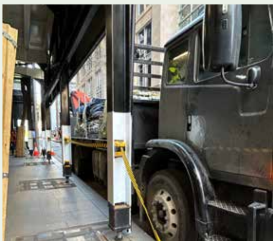
Figure 44: For public safety purposes, and subject to specific consideration by the City , approval may be given to allow the use of movable temporary concertina barriers or appropriately fitted retractable belt safety barrier systems to prevent pedestrians entering a works zone area during construction days and times.
