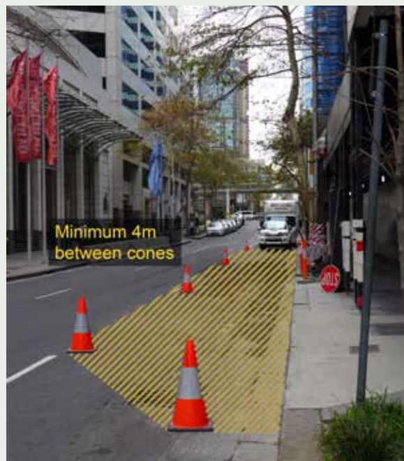
Figure 30: The use of traffic cones to delineate a works zone is not mandatory, however, where used, cones must meet prescribed requirements as set out in this Code.
