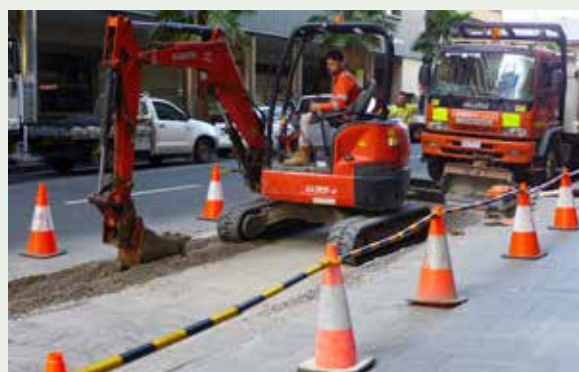
Figure 28: Road opening works must be isolated from the public accessible space by suitable barriers as determined by the PCBU or the City (where directed or required).
