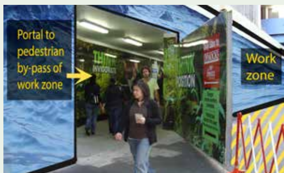
Figure 41: The hatched area indicates a works zone on a temporarily closed footway (operational only during approved works zone times). A pedestrian by-pass is available through a fully enclosed protective tunnel within a construction site.
