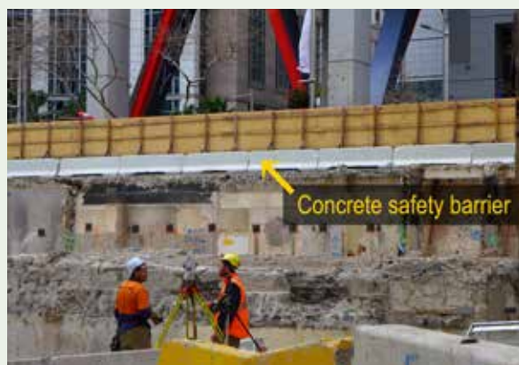
Figure 46: Excavations (deeper than 1.5 metres) must be protected by suitable barriers that the PCBU determines is required and is of an acceptable and adequate design to withstand all likely impacts including vehicular impacts.
