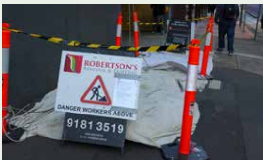
Figure 25: Exclusion zones (barricading) required by the PCBU beneath rope access hoisting activity must be of adequate stability, visibility and positioned to minimise footway obstruction. For some activities drop-sheets to protect the footway surface may be necessary or required. Where used, sheets must be placed wholly with the exclusion zone/s to eliminate pedestrian trip hazards.
