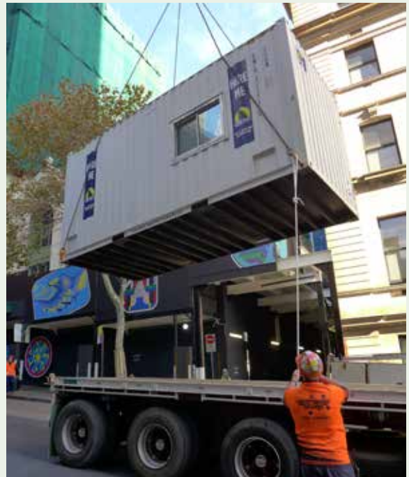
Figure 10: All hoisting operations must be carried out within the boundaries of a works zone or a temporarily closed traffic lane (to a height of at least 4.5 metres above the road surface ).
